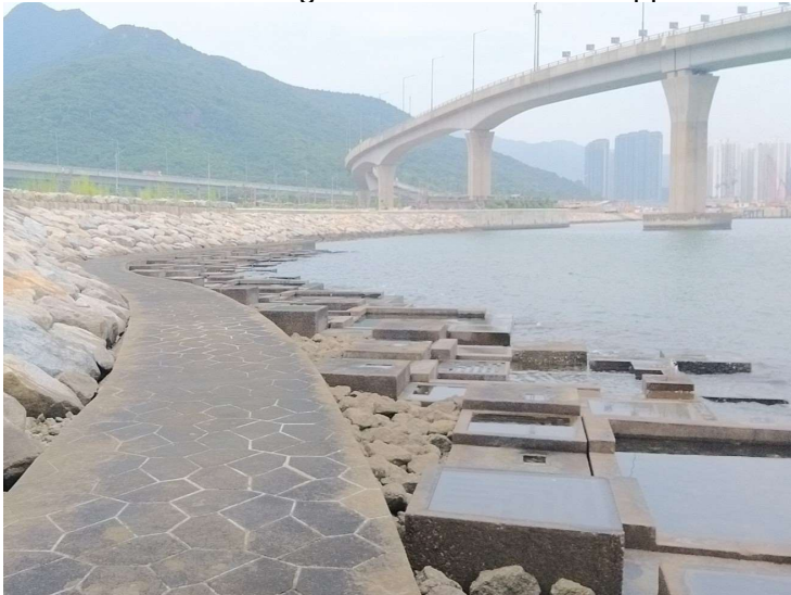
General View of Rocky Eco-shoreline
