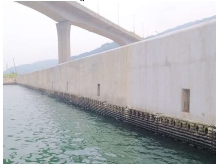
General View of Vertical Eco-shoreline
